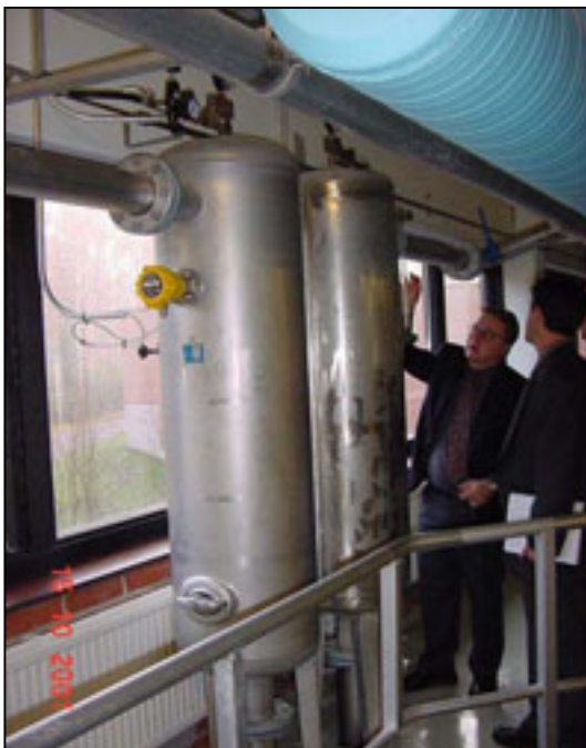
(Left & Below) A typical saturator vessel. Influent injector piece yields a high saturator efficiency, resulting in a small, compact saturator tank. All saturator MOC is 304 SS
