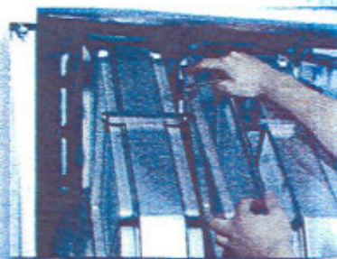
Only one fastener has to be removed to release each filter.
