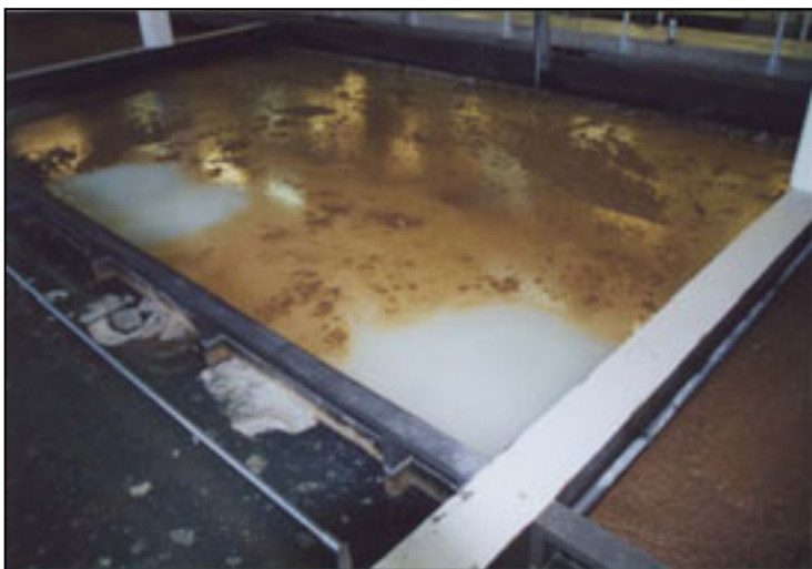
(Above) Surface of DAF basin immediately following sludge removal. (Left) Sludge clean line washes down the basin walls during sludge removal.
