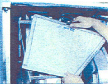
The filter basin does not have to be drained prior to the removal of filter media panels.
