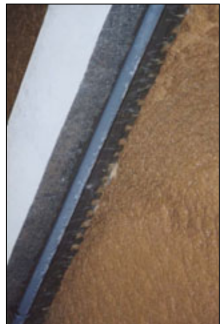
(Above) Surface of DAF basin immediately following sludge removal. (Left) Sludge clean line washes down the basin walls during sludge removal.
