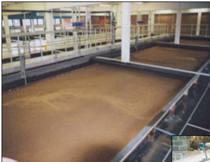
(Left) DAF basins at the Tampere WTP, Finland installation operating at loading rates of 8-12gpm/sq.ft.
